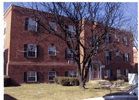
Fig. 18: OLD DOMINION WEST – Ex. Building at 3902 Old Dominion
