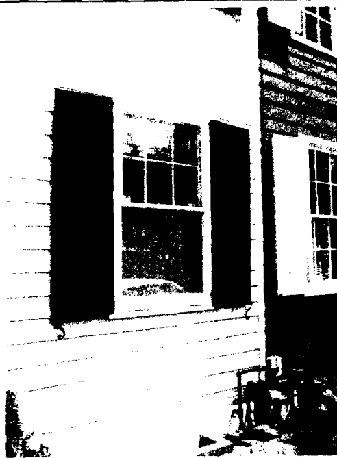
Figure 16: 2007 photograph of the same window. Notice the replaced window sill and thin sash.
