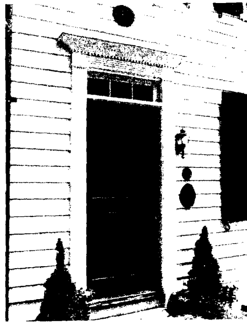
Figure 14: 2007 photograph of how the front entrance appears today. The casement around the door has been changed although the transom window remains.
