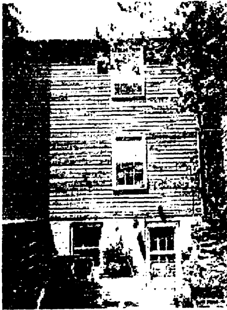
Figure 11: Rear façade showing arrangement of windows before alteration.
