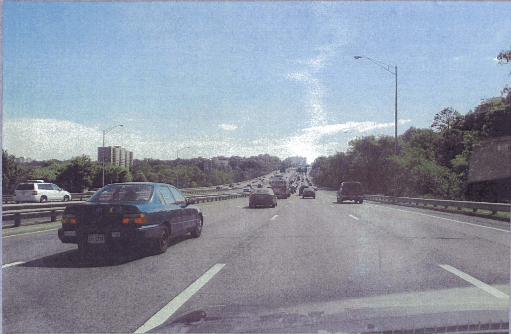
Existing View from I-395 south of Sanger Street
