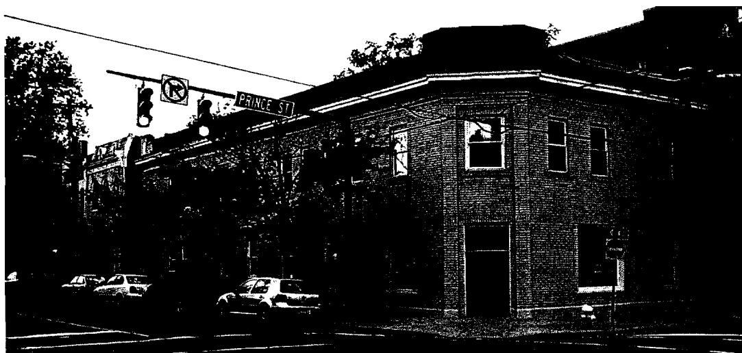
Figure 3: Photograph of 900 Prince Street after initial painting.
