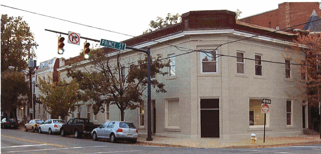
Figure 3: Photograph of 900 Prince Street after initial painting.
