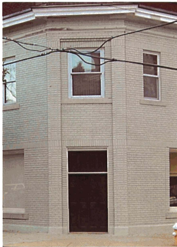
Figure 5: View of front entrance after painting showing loss of detail.
