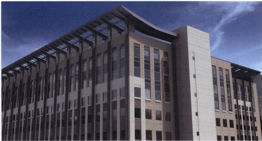
Refined Building Design with Additional Glazing and Curved Roof Canopy
