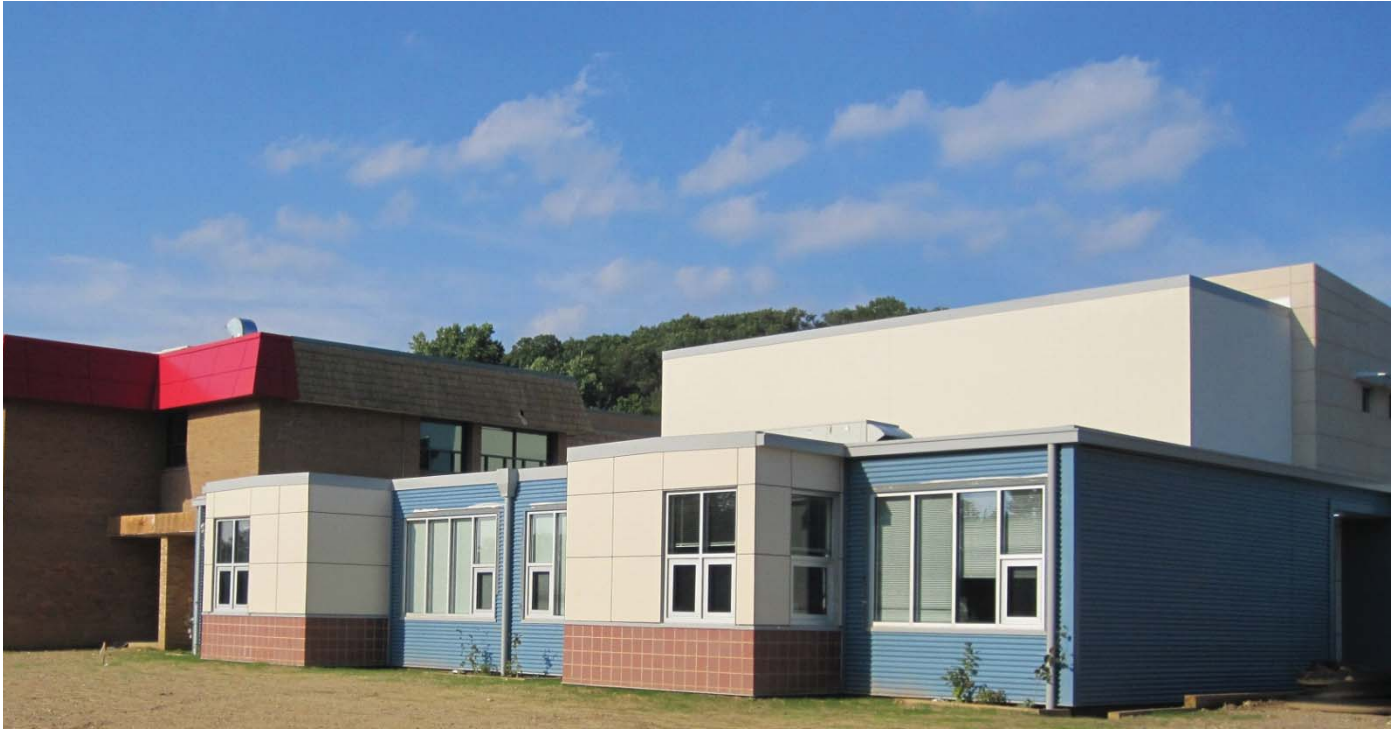
Figure 8: James K. Polk Modular Construction.
