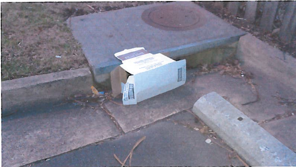
Trash blowing out of overflowing dumpsters
