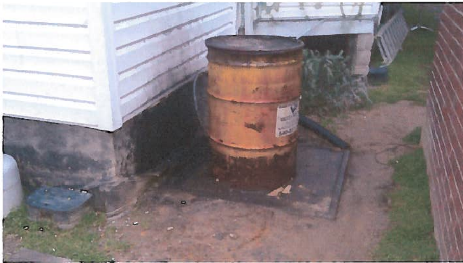
Grease barrel overflow and stains
