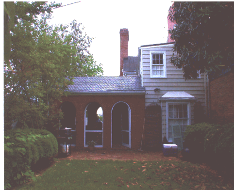
Figure 2: Existing rear view
