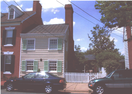
Figure 1: Existing front view
