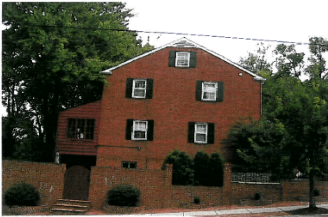
South Elevation and area proposed for demolition/encapsulation
