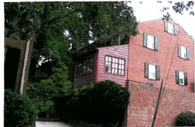
Rear (west) and side (south) elevations
