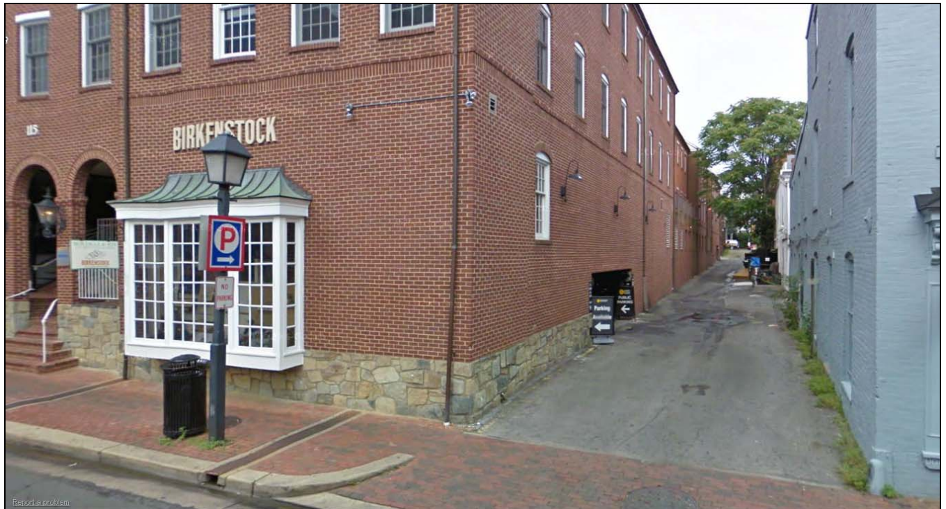
Figure 2. Existing garage entrance on South Union Street.
