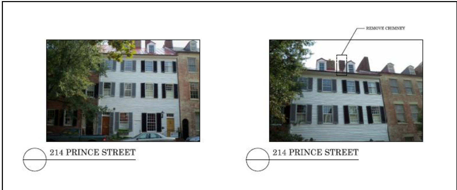
Figure 2: Proposed Chimney to be Removed
