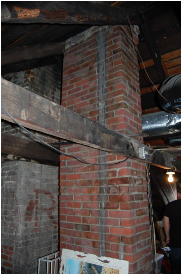
Figure 4: Attic View of Chimney to Be Removed
