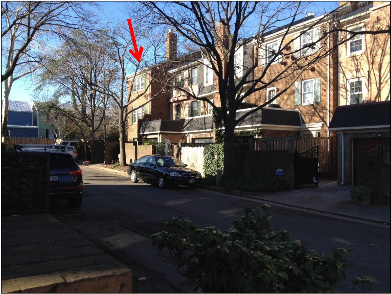
Figure 5: Existing Conditions – Alley View from N. Pitt Street
