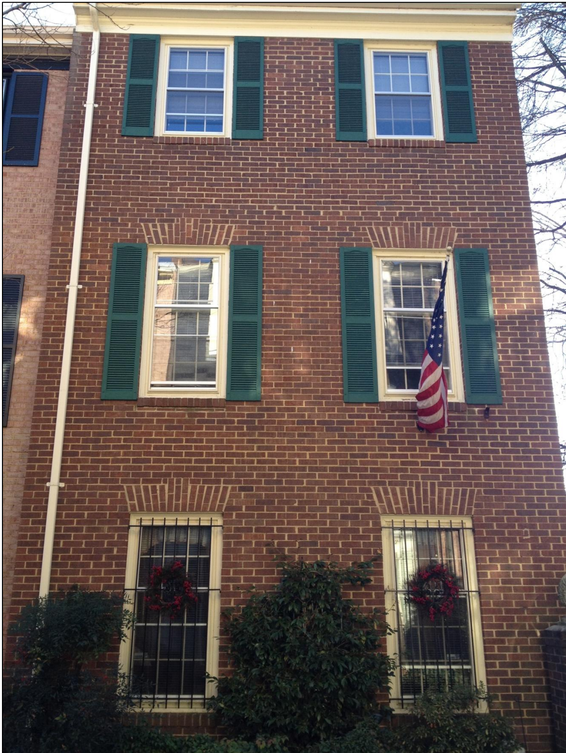
Figure 1: Existing Conditions - North Façade (Faces Courtyard)
