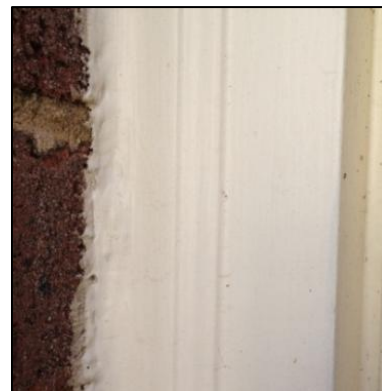
Existing wood brickmould
