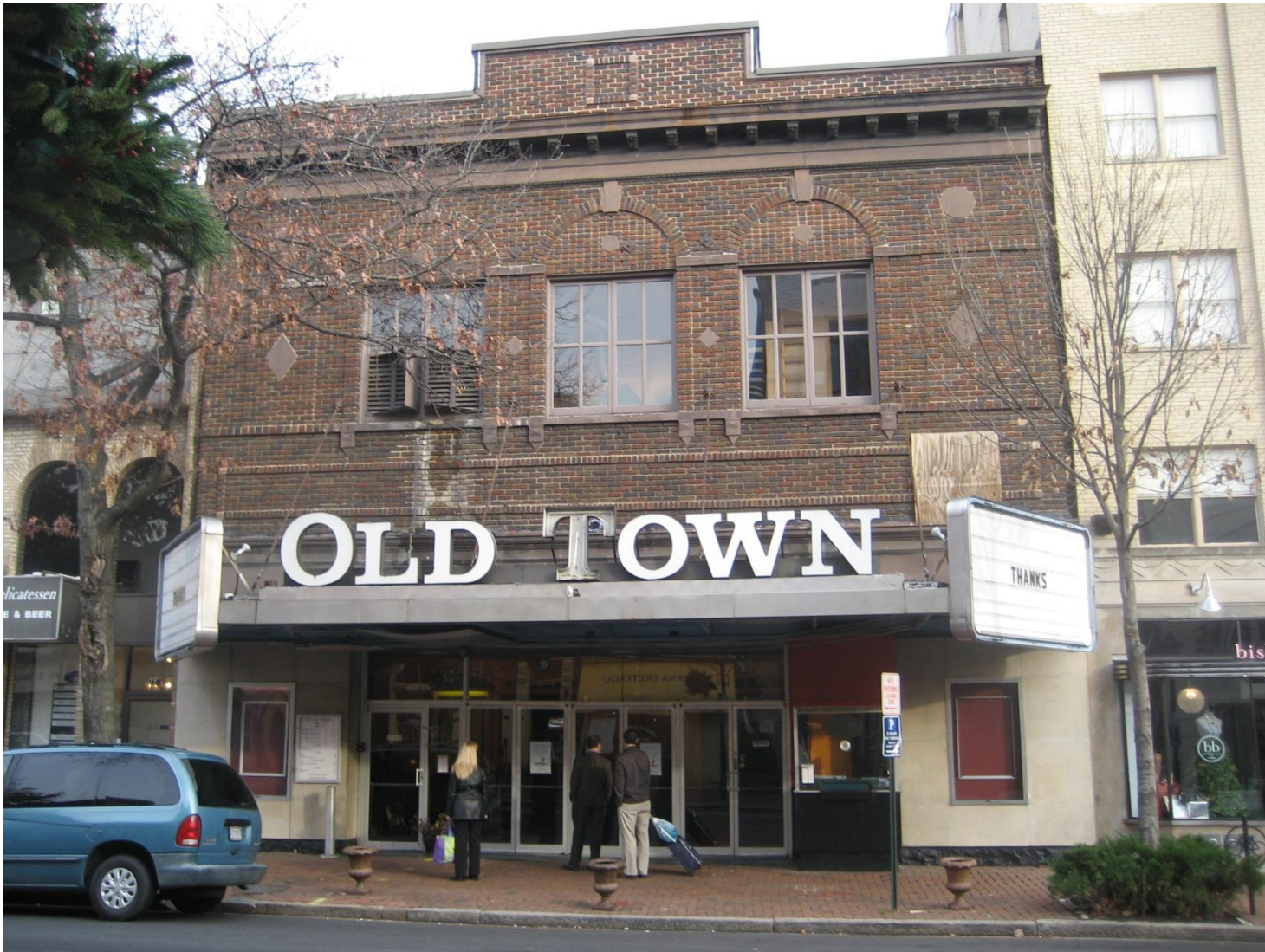
Figure 1. Existing front (south) elevation.
