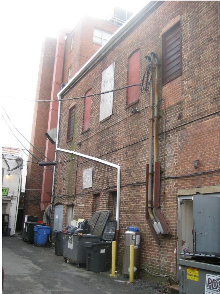
Figure 5. Existing rear (north) elevation.
