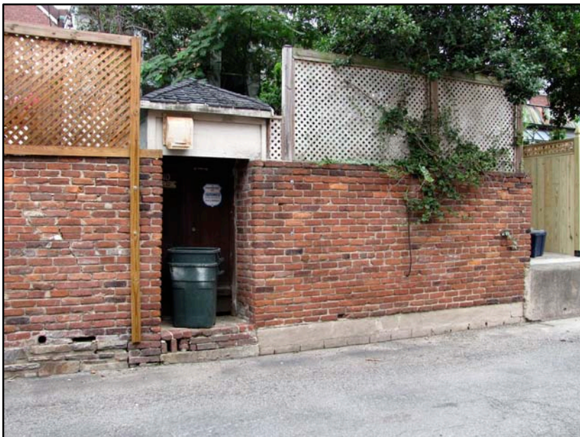
Photo 6 (showing previously existing (pre-1991) screening at 913 South Saint Asaph Street on right, and replacement screening at 911 South Saint Asaph Street on left)
