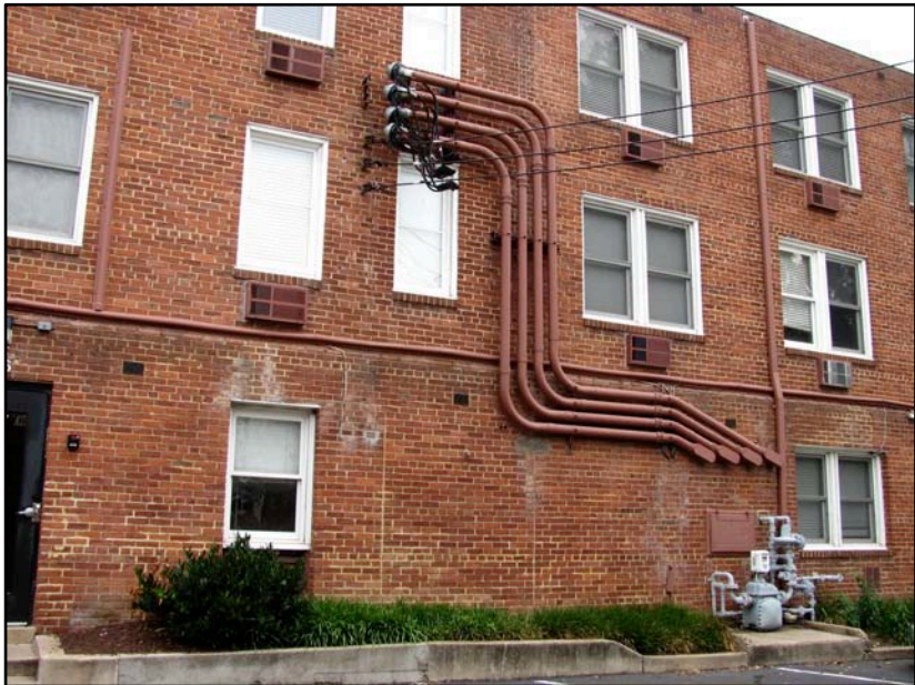
Photo 8 (showing non-conforming windows, unsightly electrical conduits, uncovered air conditioning unit, unscreened utilities)
