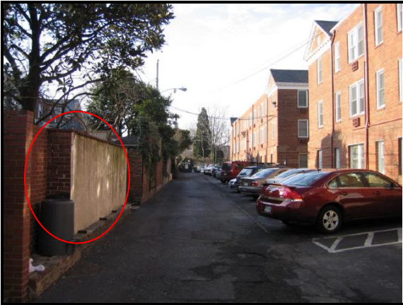
Wall condition in May 2009
