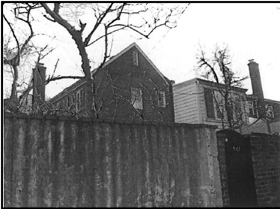
Wall condition in May 2009
