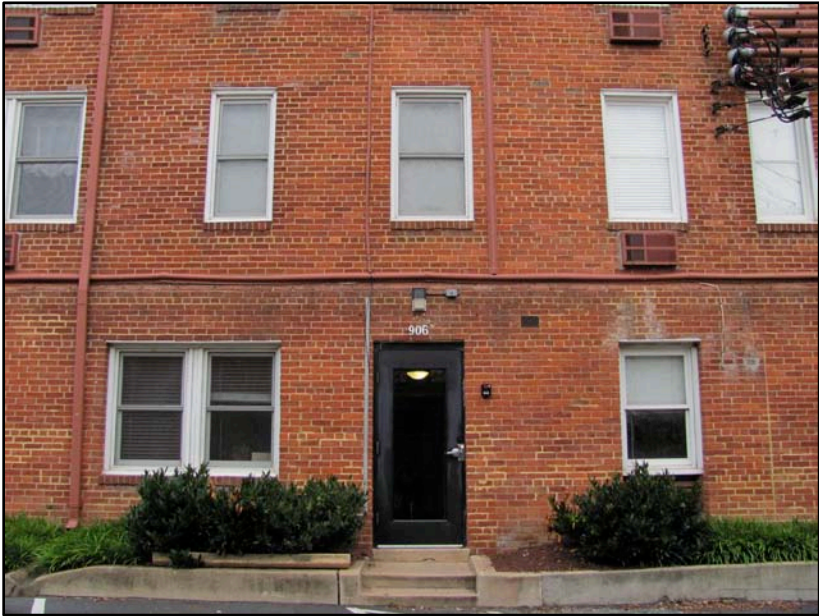
Photo 7 (showing rear entrance to the Bearings condominiums, spotlight above door, non-conforming windows, overhanging air conditioning units, unsightly exposed electrical conduits and wiring)
