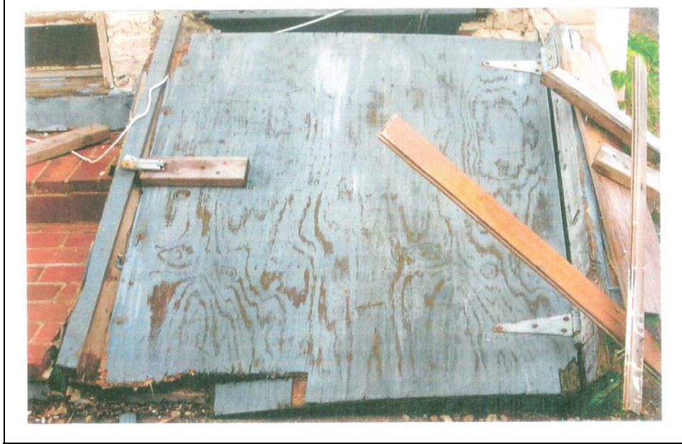
Figure 7: Existing basement hatch
