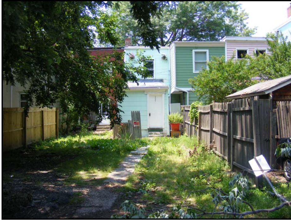
Figure 4 Existing Rear Elevation
