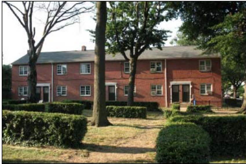
Figure 4. Existing building on North Patrick Street.
