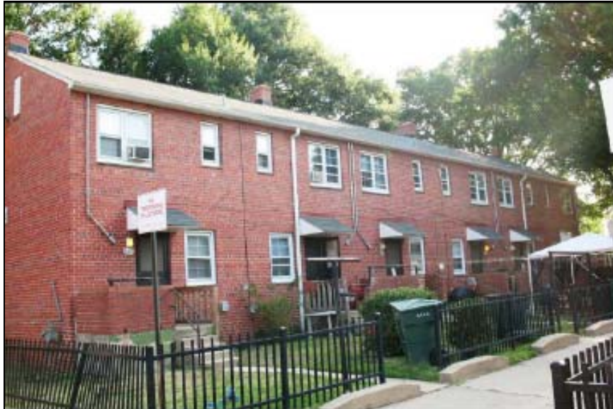
Figure 7. Existing building on North Alfred Street, illustrating typical rear elevation.
