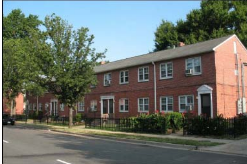
Figure 6. Existing building on Madison Street illustrating typical front elevation.
