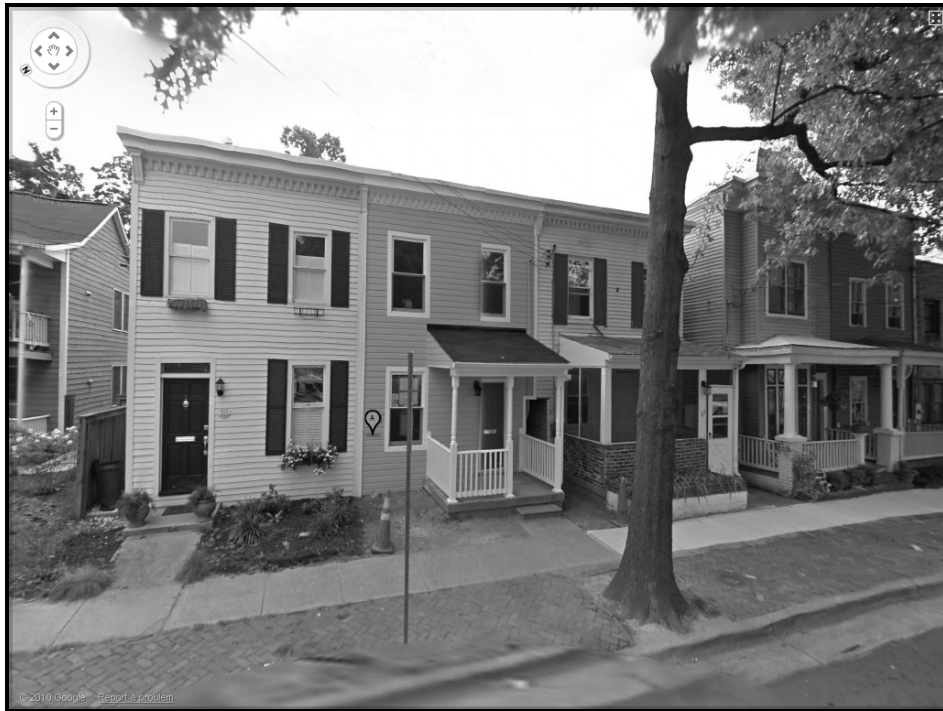
Figure 2. Photo of Existing Conditions – Front Elevation
