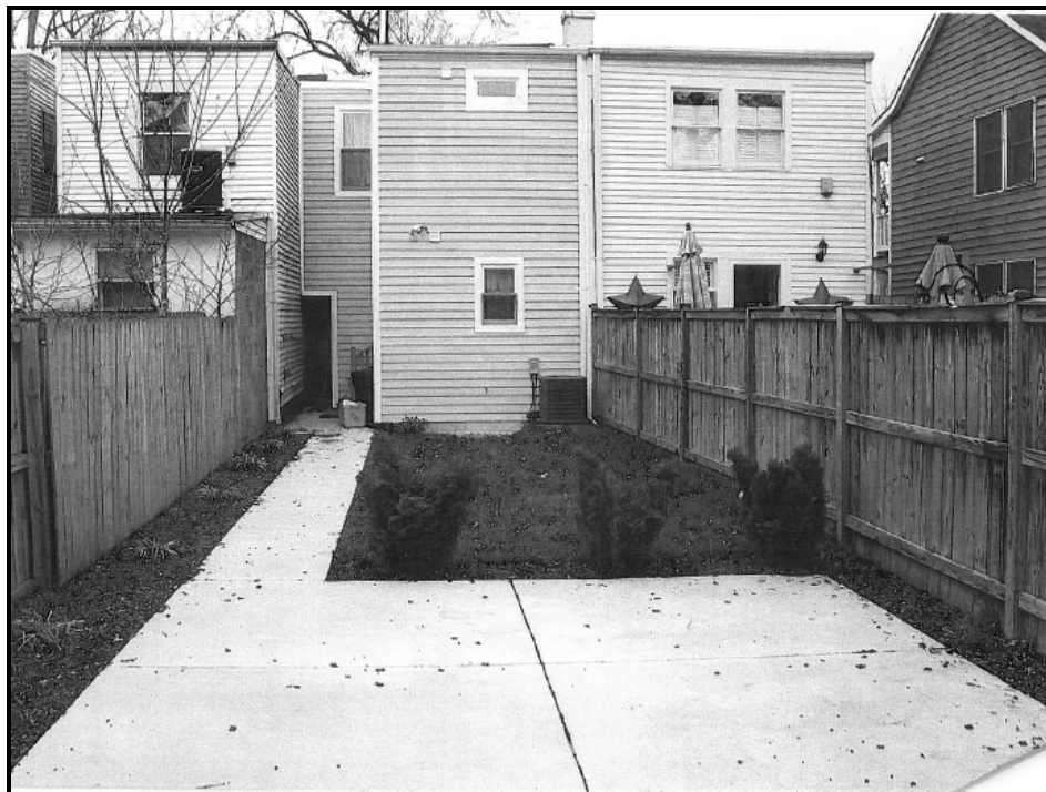
Figure 3. Photo of Existing Conditions - Rear Elevation
