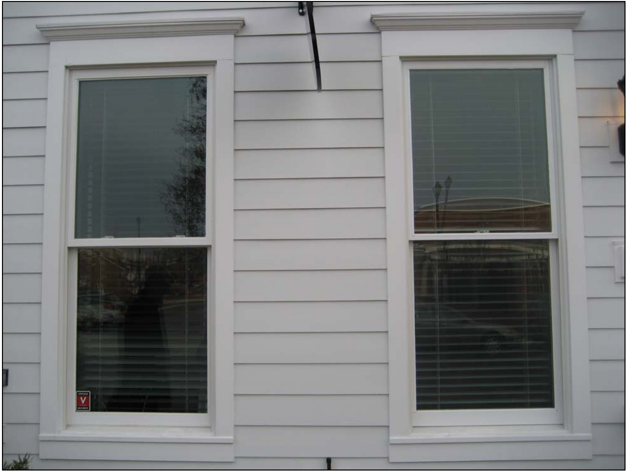
Figure 1. Model unit, 735 North Columbus Street, with painted CPVC window on left and painted wood window on right.
