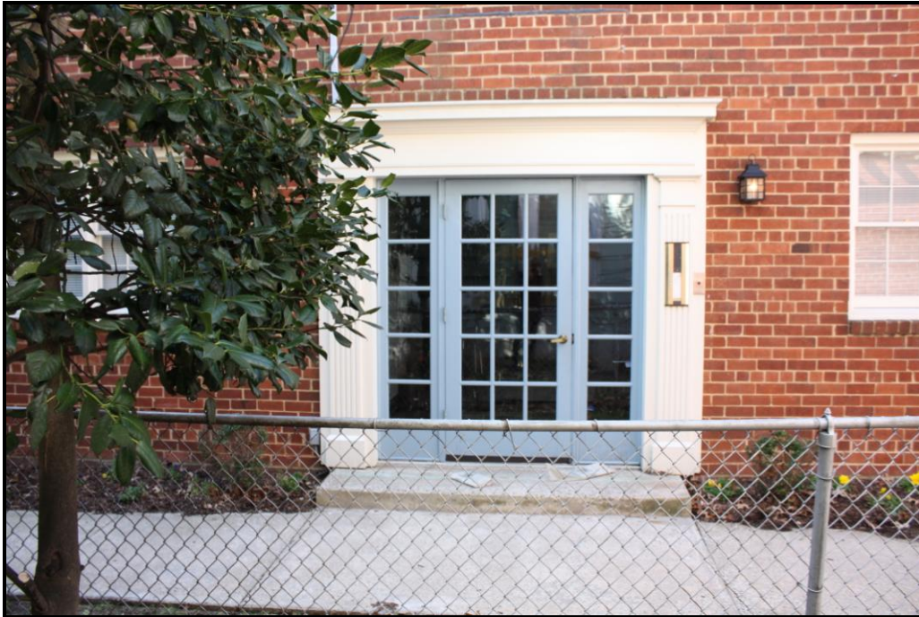
Figure 6: View of Front Entrance of Adjacent Building
