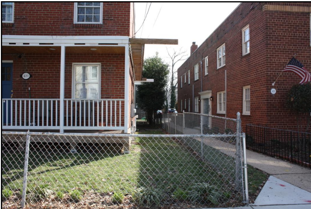
Figure 5: View of Front Elevation and Adjacent Building
