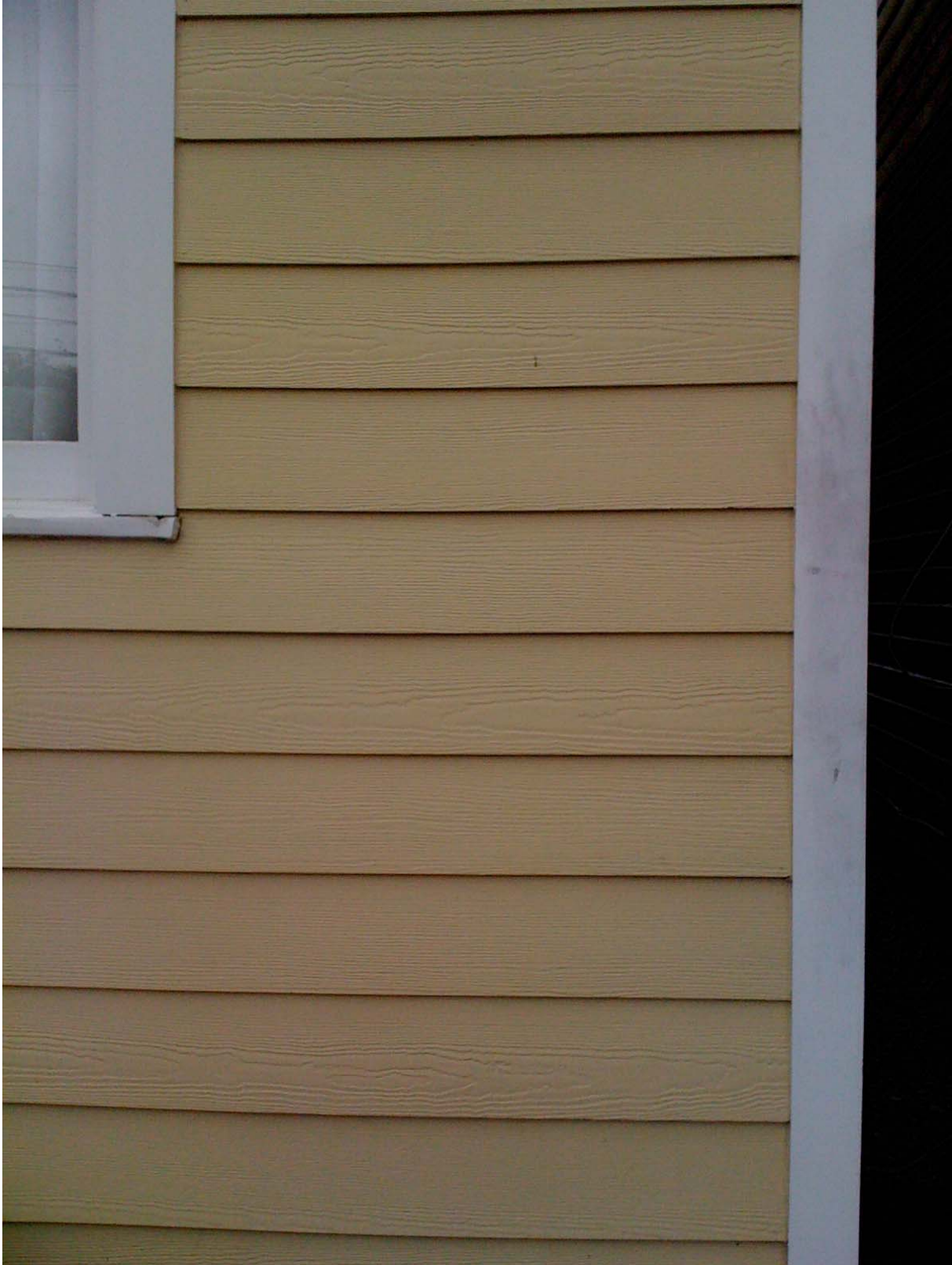
Figure 7: Existing Fiber Cement Clapboard Siding With Wood Grain Pattern
