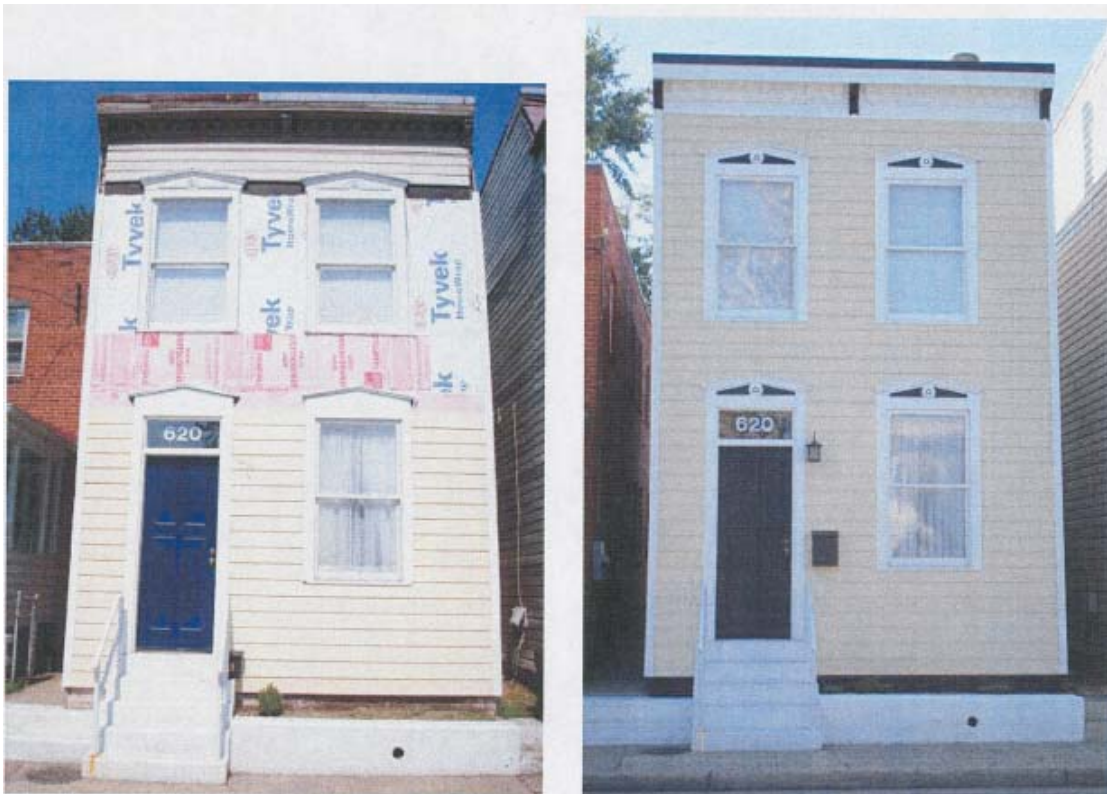
Figure 2: Photo of Front Elevation of House (After installation of HardiePlank)
