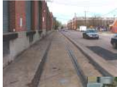
Figure 6: Existing Rail Line on N Fayette St
