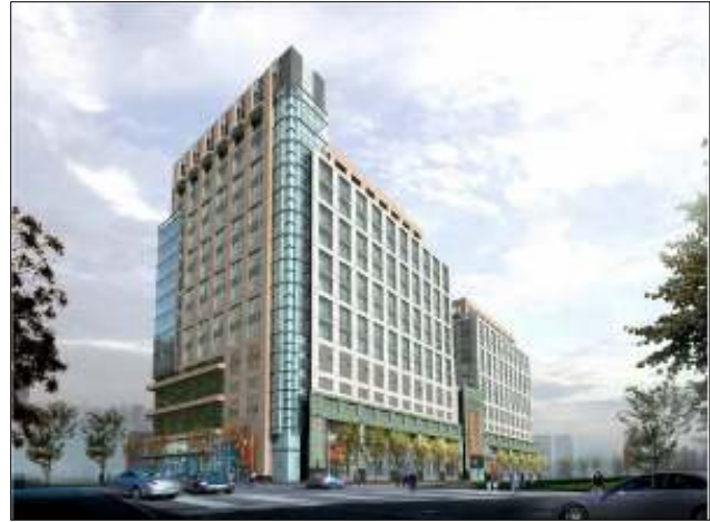
Figure 12: Block P Building Top
