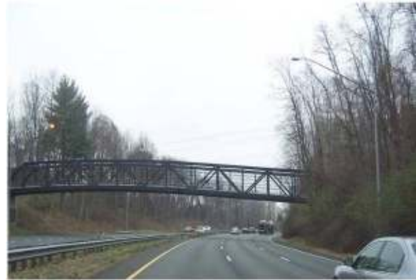
Figure 5: Bridge at Capital Crescent Trail
