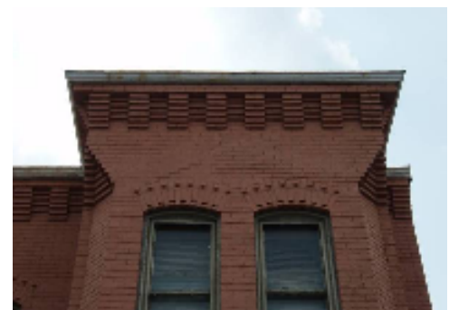
Figure 15: Building Details on Washington Street
