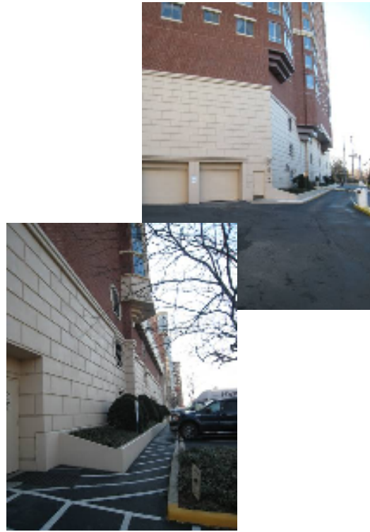
Figure 21: Existing Sidewalk Adjacent to High-Rise Buildings
