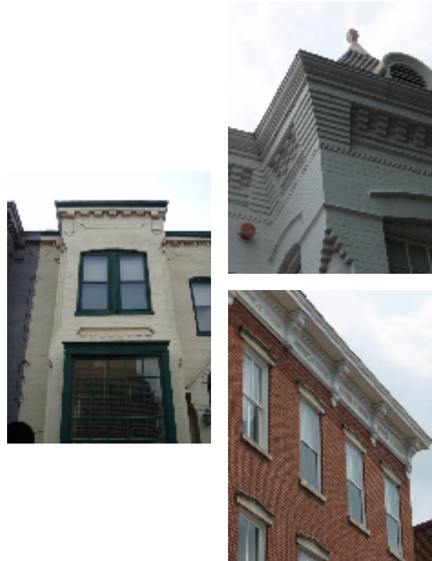
Figure 4: Building Details on Washington Street
