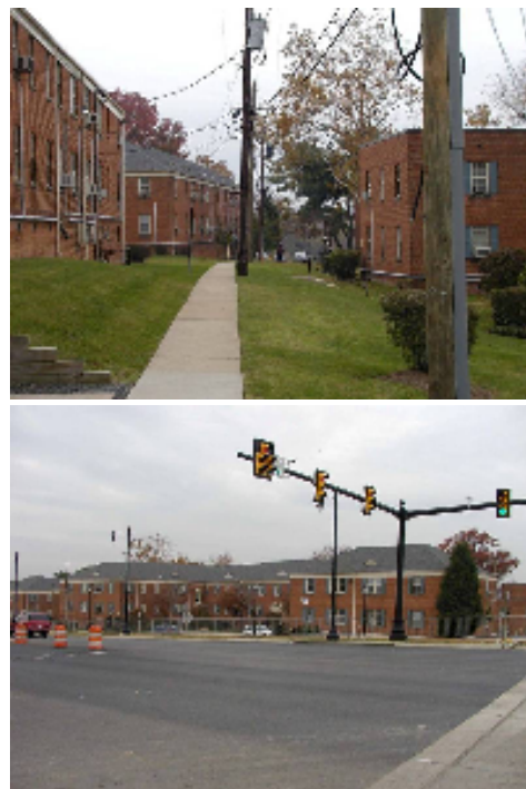
Figure 8: Existing Hunting Terrace Apartments
