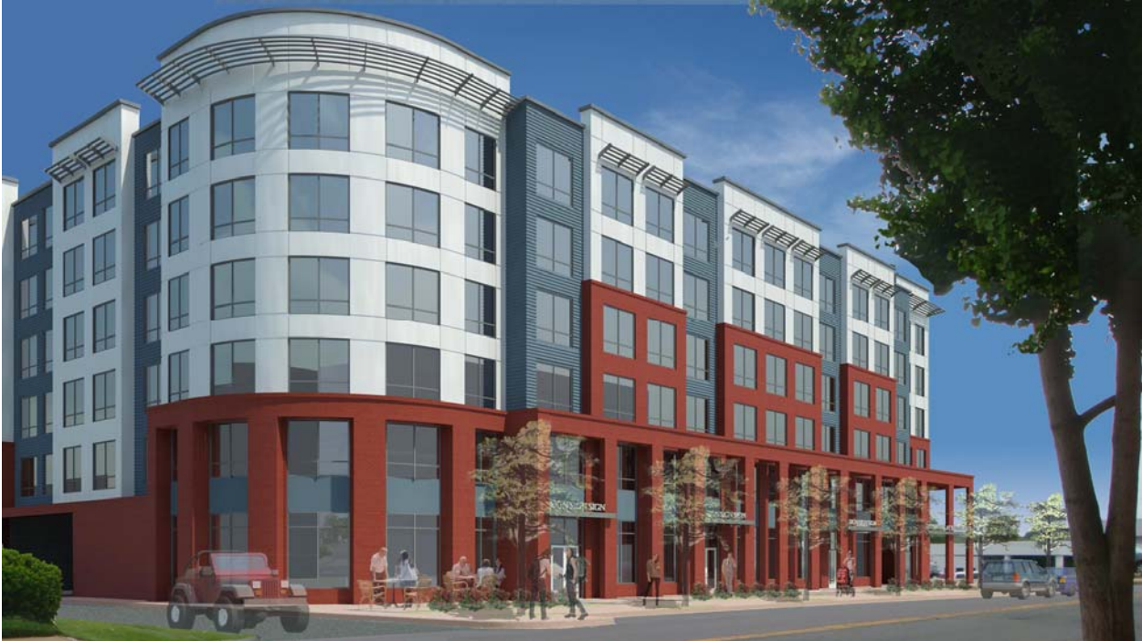
View of building looking southwest
