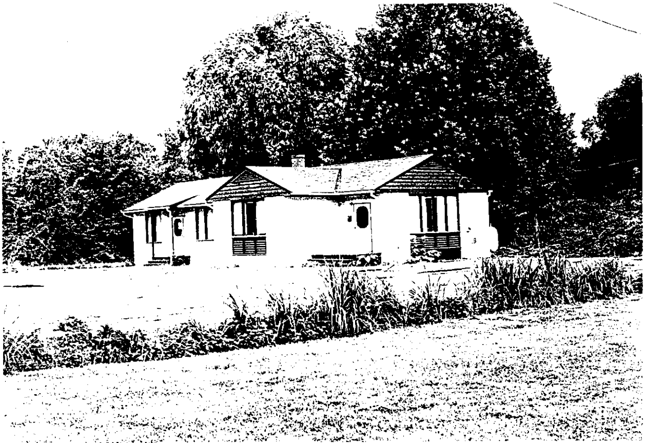
Existing Seaport Foundation workshop north of bridge to be demolished
