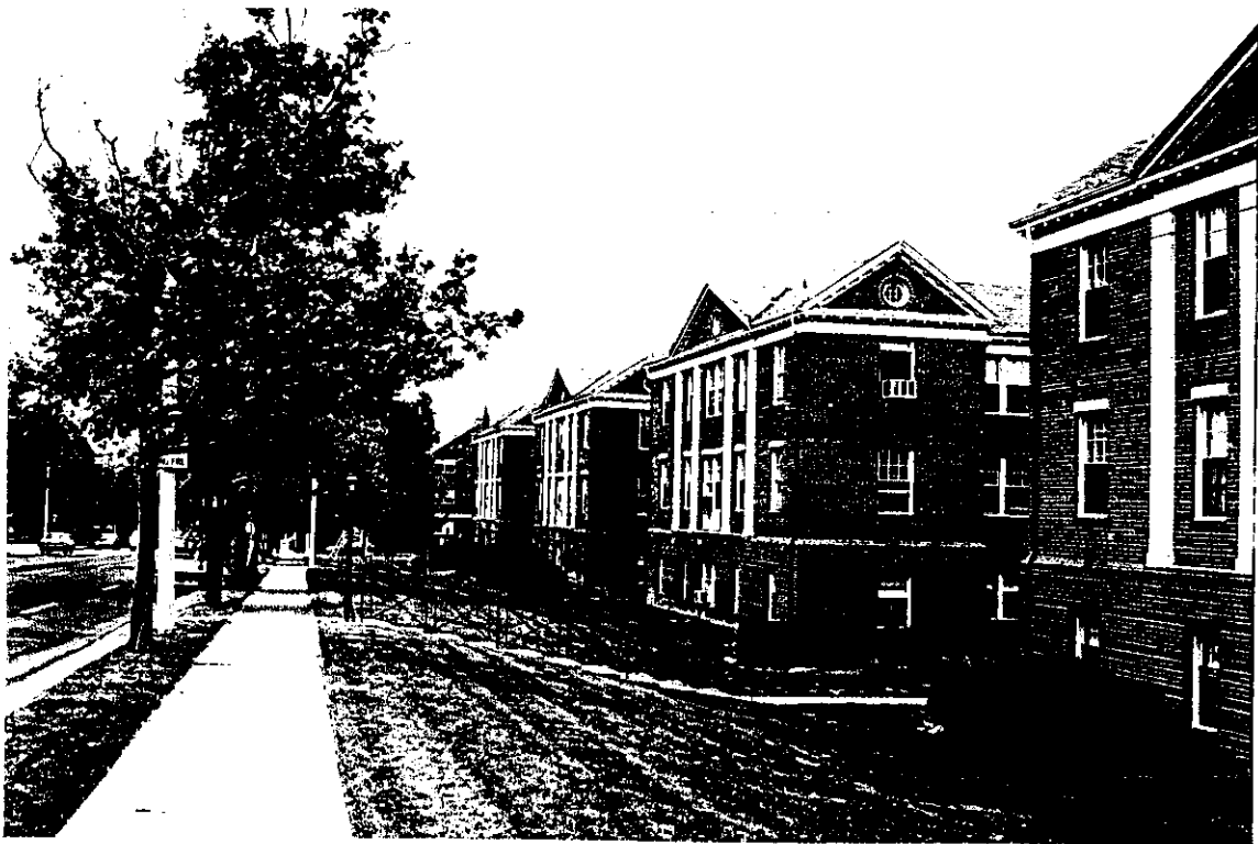
Residential buildings on Washington Street north of the proposed deck-over showing existing street trees and building setback
