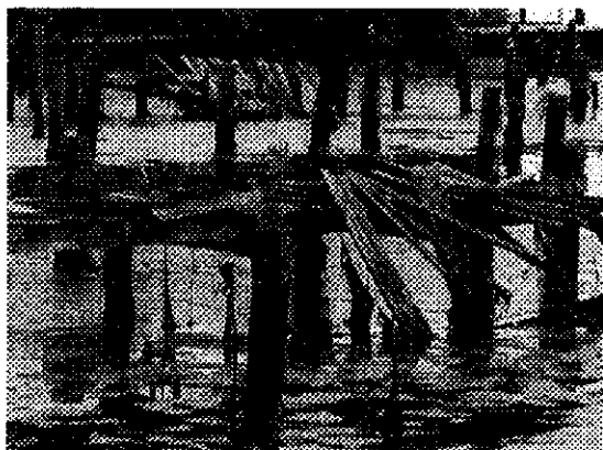
Plate 3.6: View of the decaying pilings.
