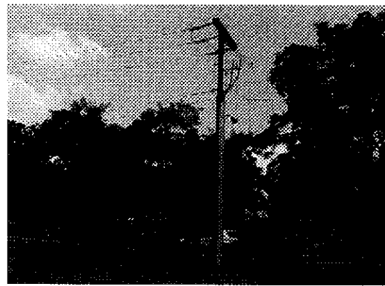
Plate 3.9: Existing overhead power line along Union Street.
