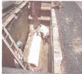
Interceptor Rehabilitation Project on Commonwealth Avenue
