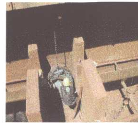
Rehabilitation of Existing Sand Filter
