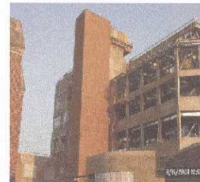
On-going Construction of Solids Handling Building
