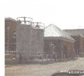
Construction of Methanol Addition Facilities
