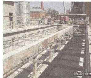
Construction of New Secondary Settling Tank #5
