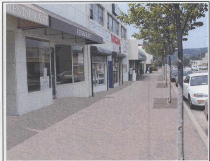
Brick pavers where missing
