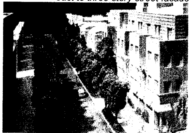
Three story façade on street. Two stories of office over retail
