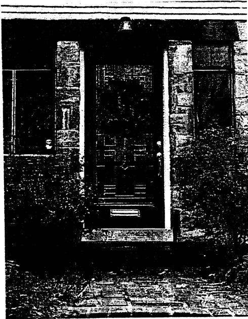
Figure 1 The new front door as installed at 1302 Michigan Avenue
