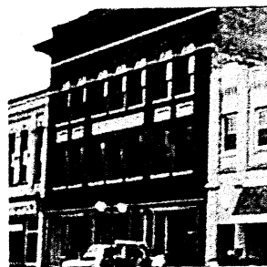
Example of Artists' Loft Building, Artspace Projects Inc.
