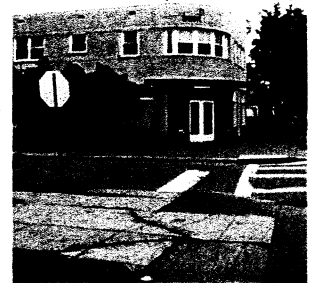
Poor quality pavers
