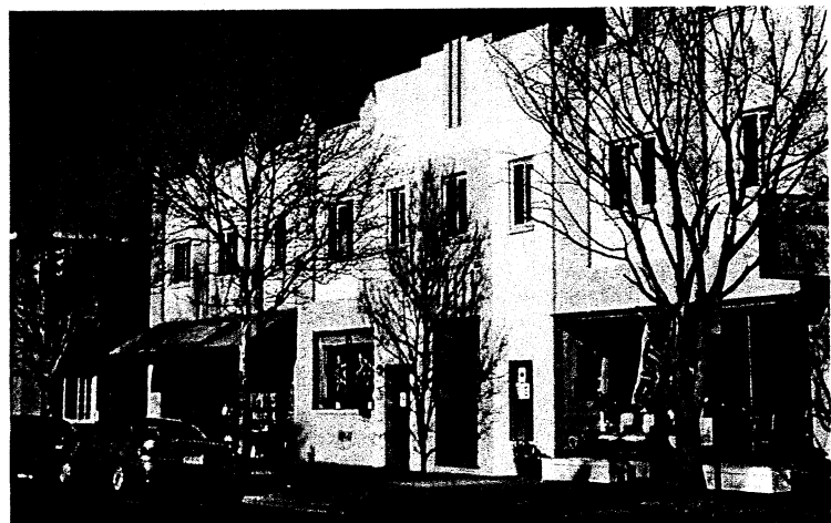
Figure 6.16 Architectural detail and interest
