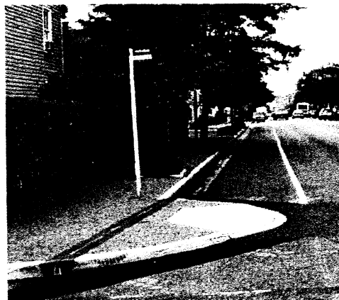
Example of Existing Bulb-out
