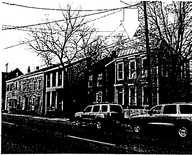
Figure 1 - View north on Patrick Street with subject property on right
