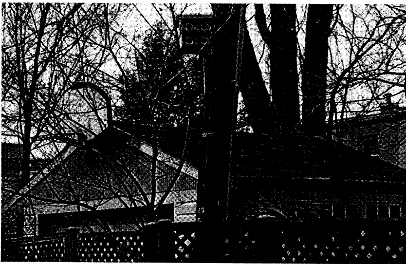
Example of metal clad garage in 100 block of North Peyton Street
