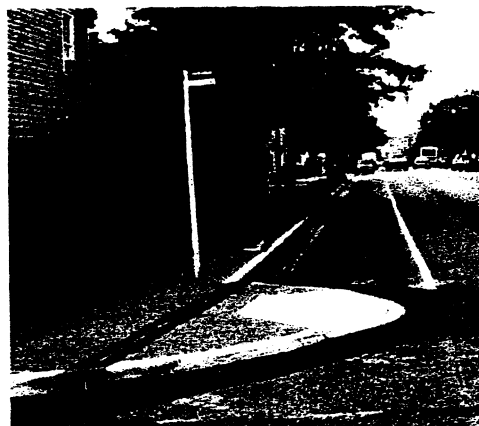
Example of Existing Bulb-out
