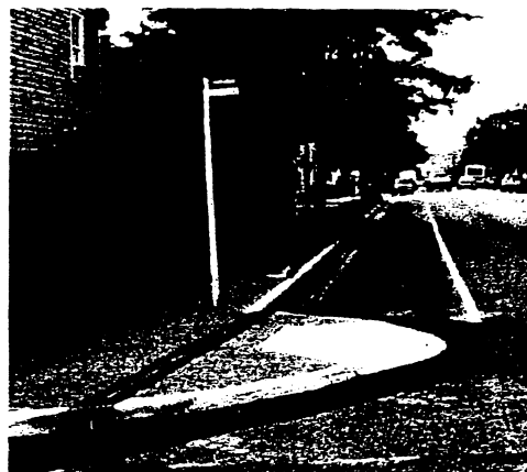
Example of Existing Bulb-out
