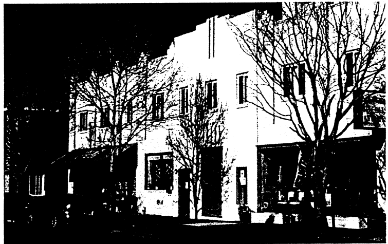
Figure 6.16 Architectural detail and interest
