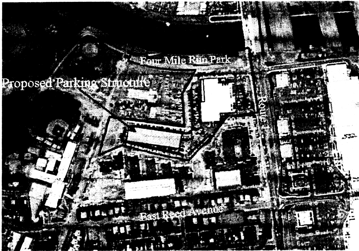
Aerial View of Site with Proposed Parking Garage and Service Bay Additions
