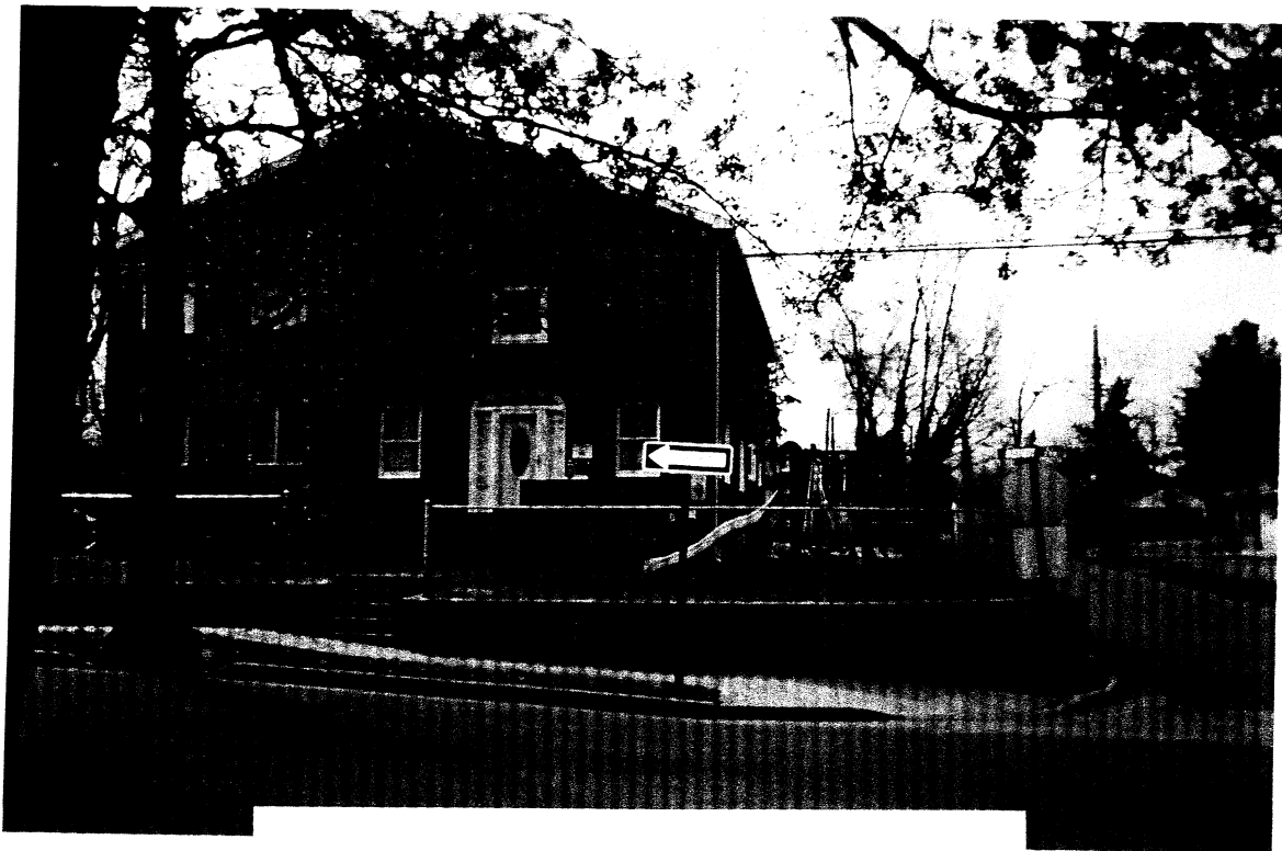
201 SE corner of Ashby and Wilson 12ft side yard 26ft height
