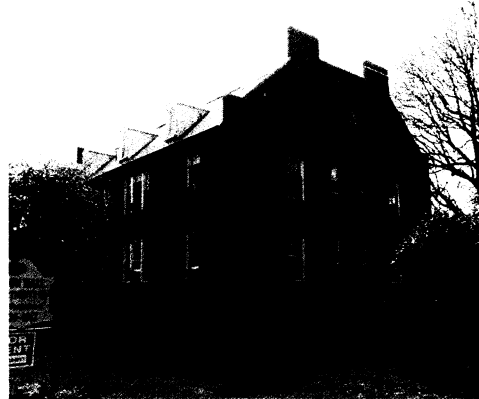
Figure 5 Gunston Hall Apartments, designed in a conscious Colonial Revival style in 1939, employs many of the same design elements as the original Gunston Hall plantation building including brick construction, slate covered gable roof with dormers, double chimneys, pedimented door surrounds quoining and circular windows.
