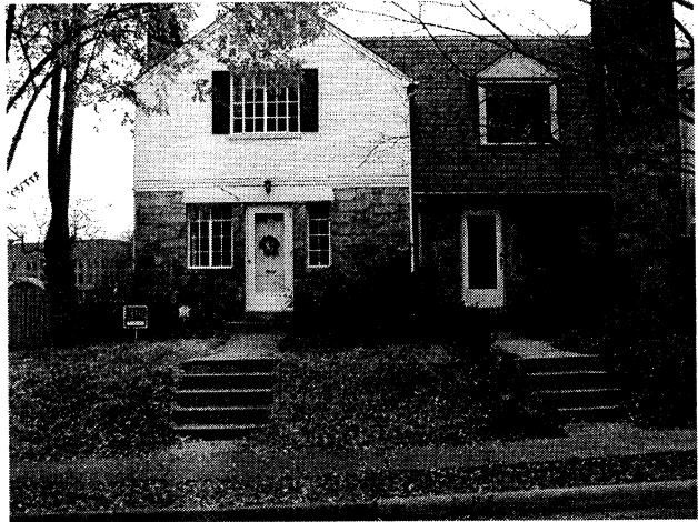
Figure 2 Appropriate front doors as installed in the development
