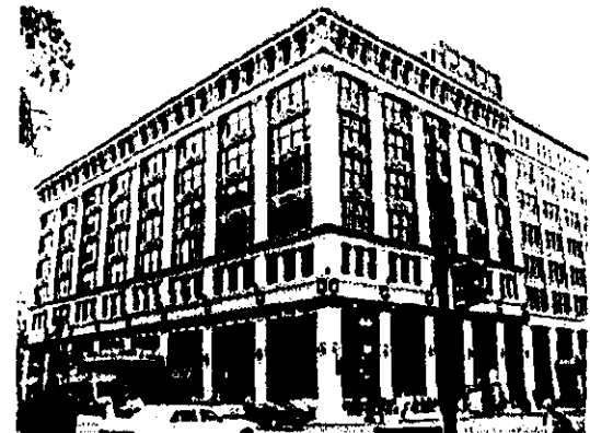
An example of an approximately 5-story base building
