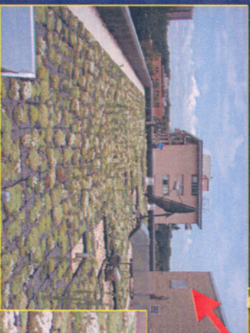
Re-vegetated modules were installed over foam matting and filter fabric.
