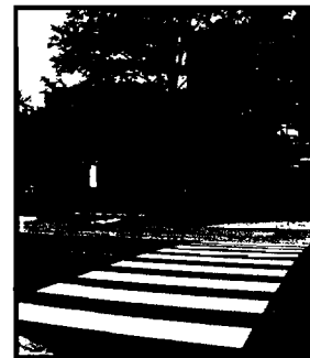
Figure 11. High-visibility Thermoplastic Crosswalk
