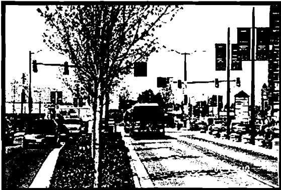
Fig. 3. Median transitway in Vancouver, BC
