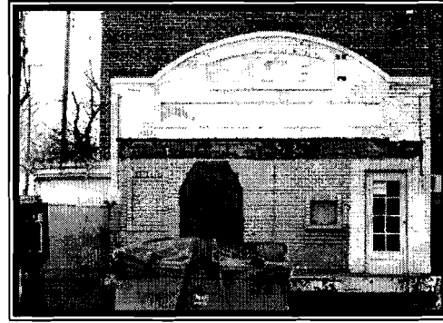
Figure 3 - Ice House after demolition of the canopy
