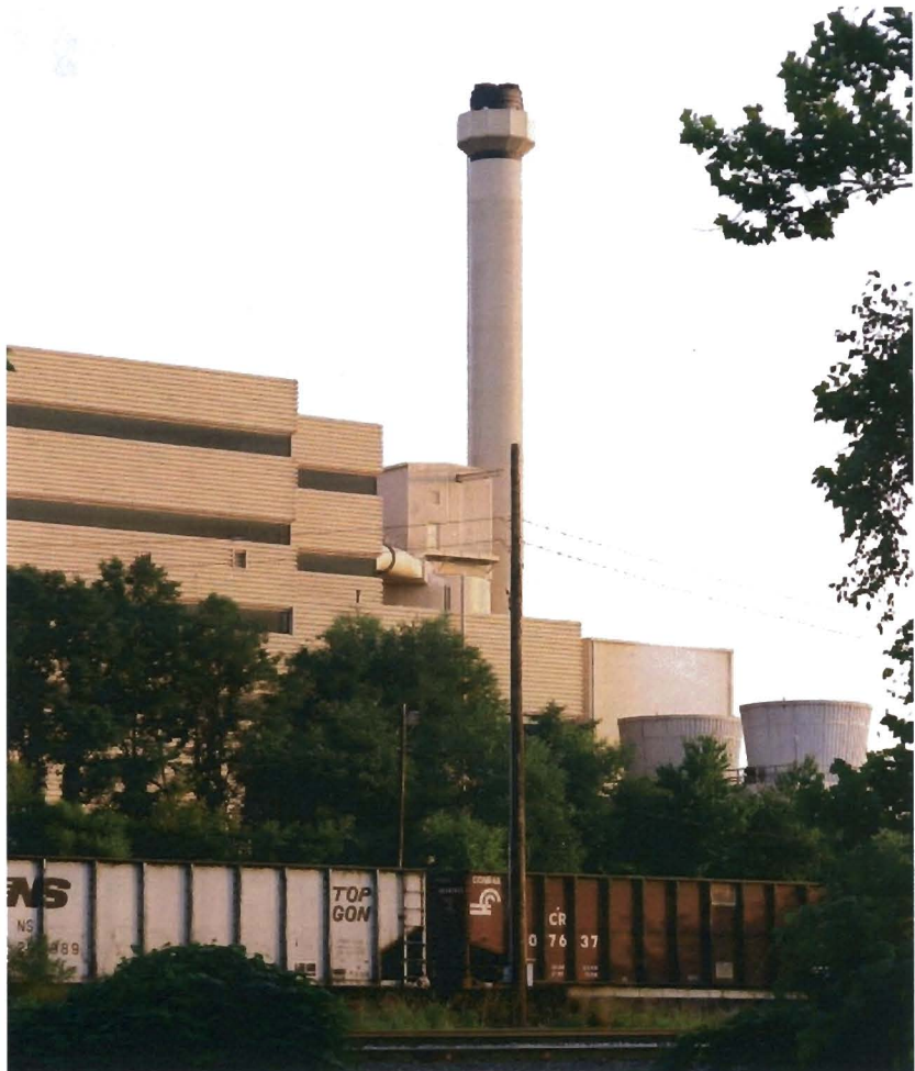
The Covanta Energy-from-Waste Facility supplies enough electricity to power approximately 20,000 homes in Northern Virginia.
