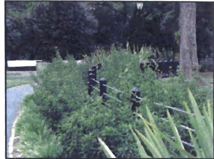
Figure 7. Post and Cable Security Fencing
