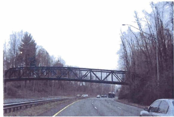
Figure 5: Bridge at Capital Crescent Trail
