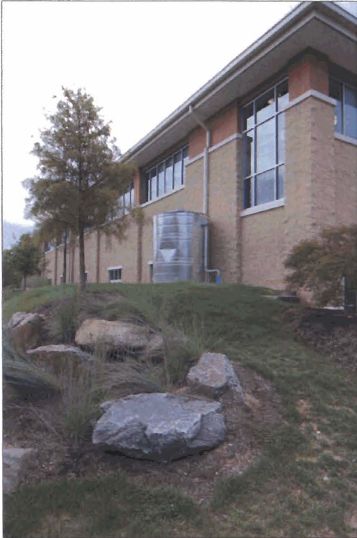
Figure 8-5. Cisterns For Greywater Re-use, Arlington, VA
